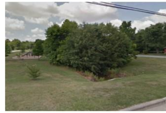
Drainageway 68 Greensboro, NC
